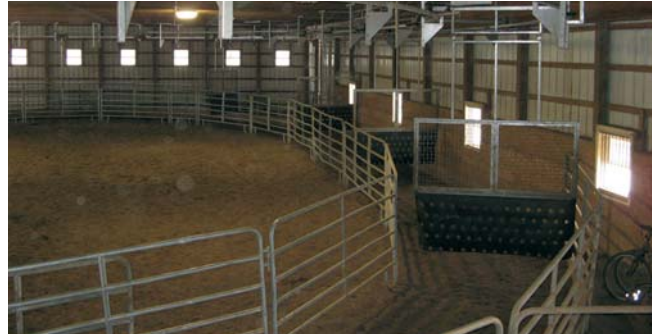
Rail-Gliding Horse Walker, Oval 15 x 30m (50'x99') for 12 horses installed in an existing building. Bookman Stables, Acron, Ohio, USA
