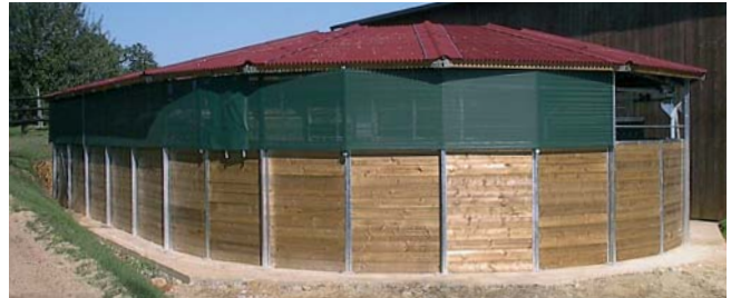
Fence Type D : horizontal spruce boards, 40 mm (1.5") thick x 2 m high (6.5'), with edge protector (widths vary)
