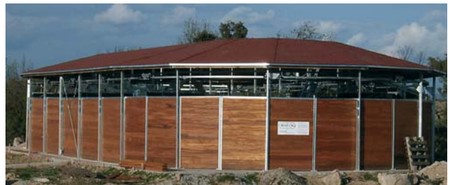
Fence Type E : horizontal hardwood boards, 40 mm (1.5") thick x 2 m high (6.5'), with edge protector (widths vary)
