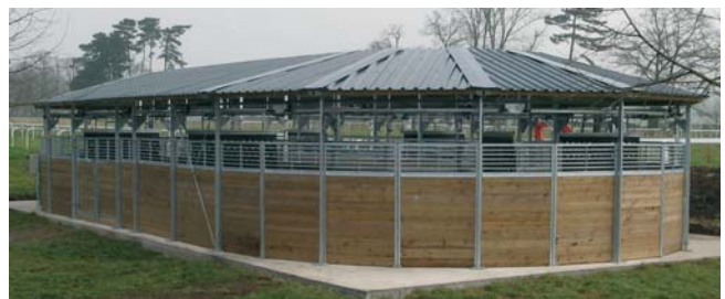
Fence Type F : horizontal spruce boards, 40 mm (1.5") thick x 1.5 m (5') high, (widths vary) with galvanized, framed welded wire grid from 1.5 to 2 m (5' to 6.5') high
