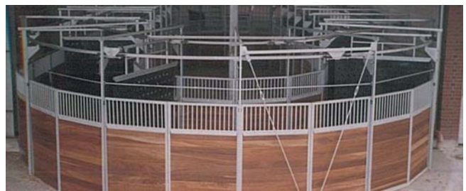
Fence Type G : horizontal hardwood boards, 40 mm (1.5") thick x 1.5 m (5') high, (widths vary) with galvanized, framed welded wire grid from 1.5 to 2 m (5' to 6.5') high
